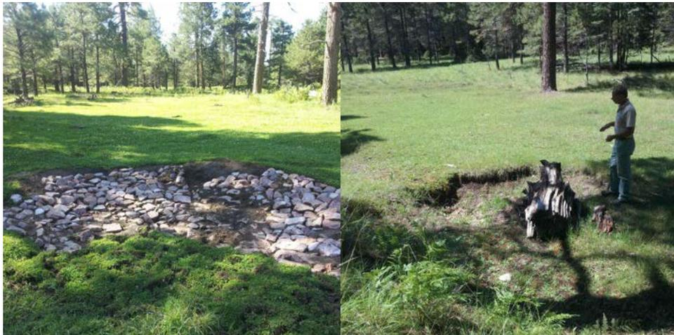
The picture on the left is a completed Zuni Bowl. The picture on the right is one of the down cuts at Holder Cabin that would be repaired in 2013. Note the steep bank on the upstream side of the bowl. This steepness allows for rapid head cutting and down cutting, both great adverse impacts to the hydrology of these important meadows.
